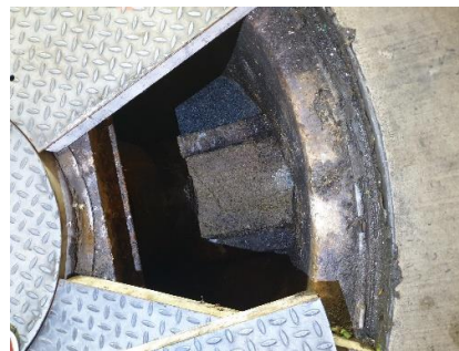
Inspection and sampling at premises
